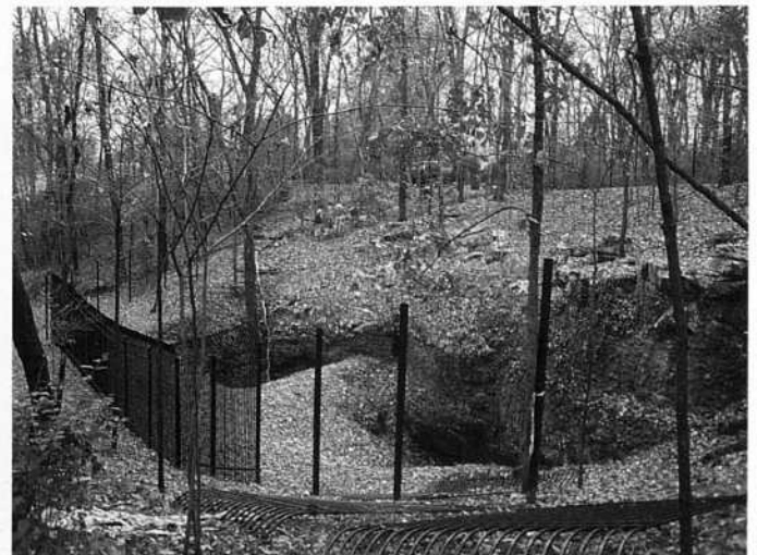
Southern side of fence nearly completed
